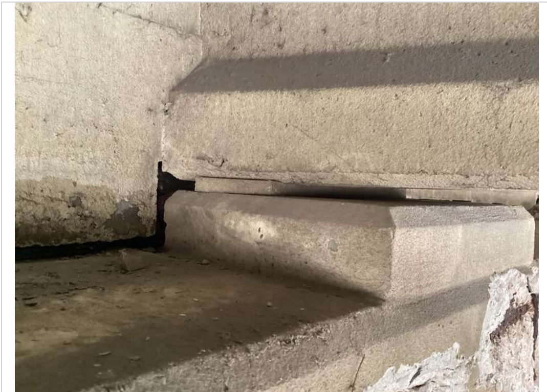
Abutment 2 bearing typ
