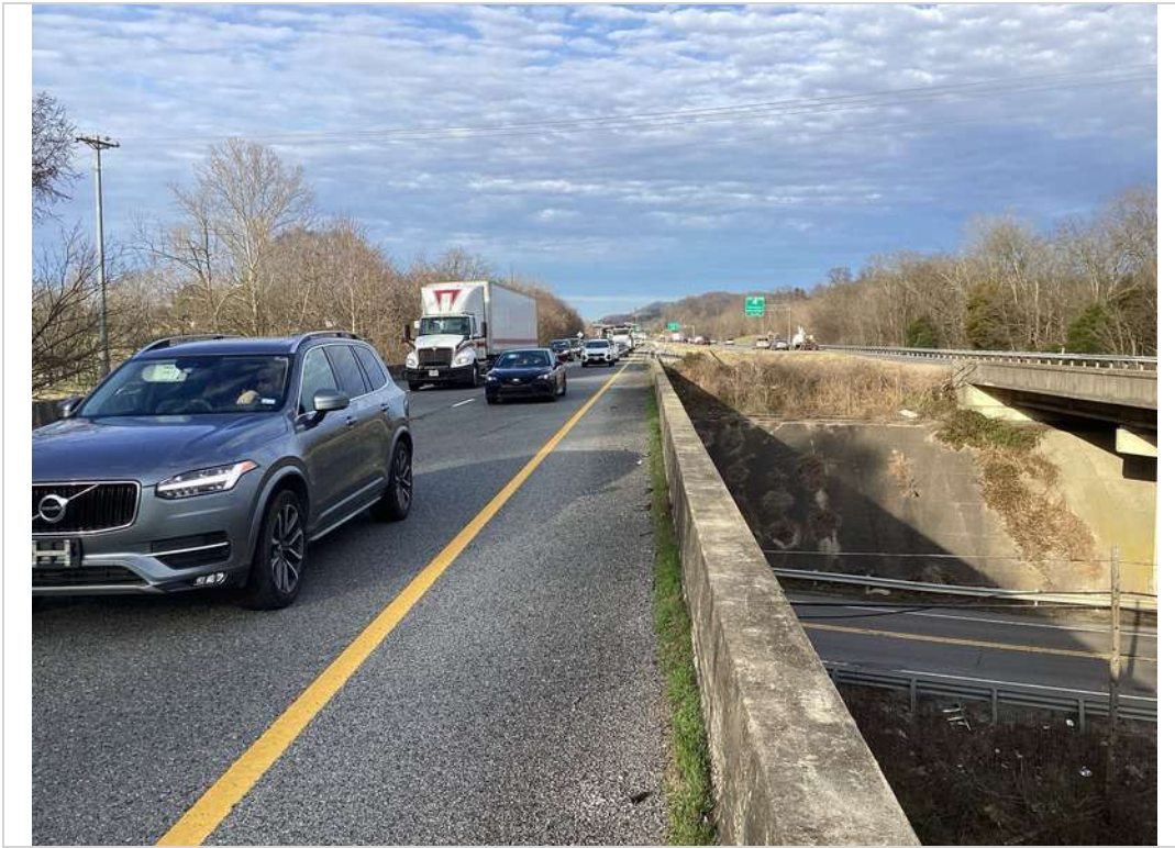
Top of deck looking forward
