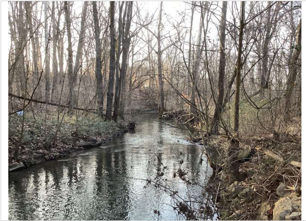
Looking downstream from beneath bridge
