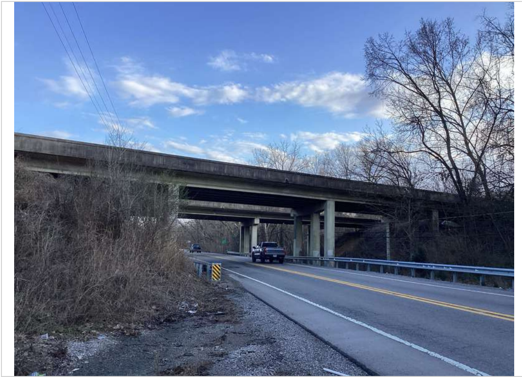
Downstream left side elevation
