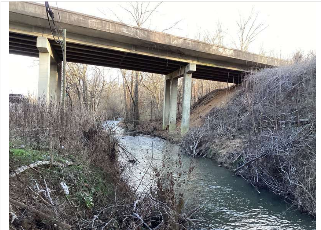
Looking upstream from beneath bridge
